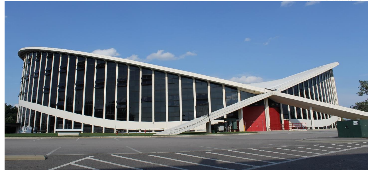
Dorton Arena West Side
